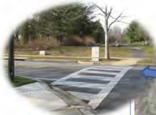
Photo 2. A curb extension and high visibility crosswalk such as this are recommended for the school entrance.
